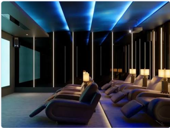
A Casambi lighting setup — lights, shades and appliances, all controlled from Control4 Navigator and the Control4 app.
